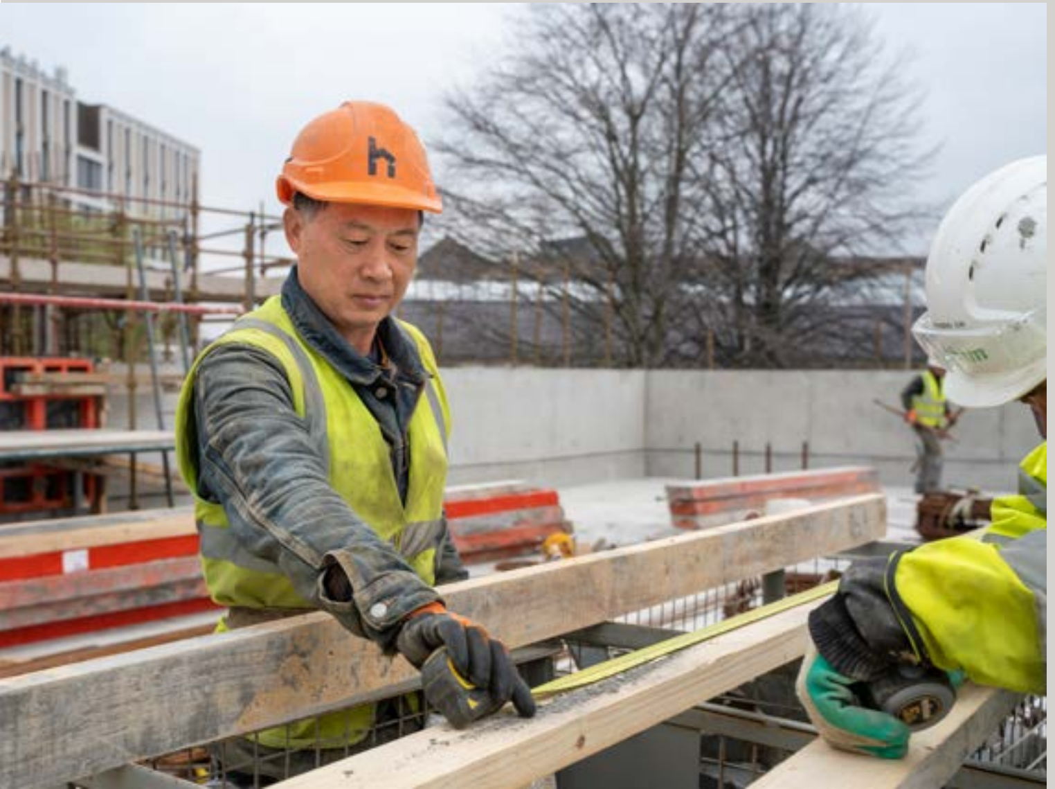
Construction workers on the D7ET School site, March 2022. Image: Conor Mulhern
