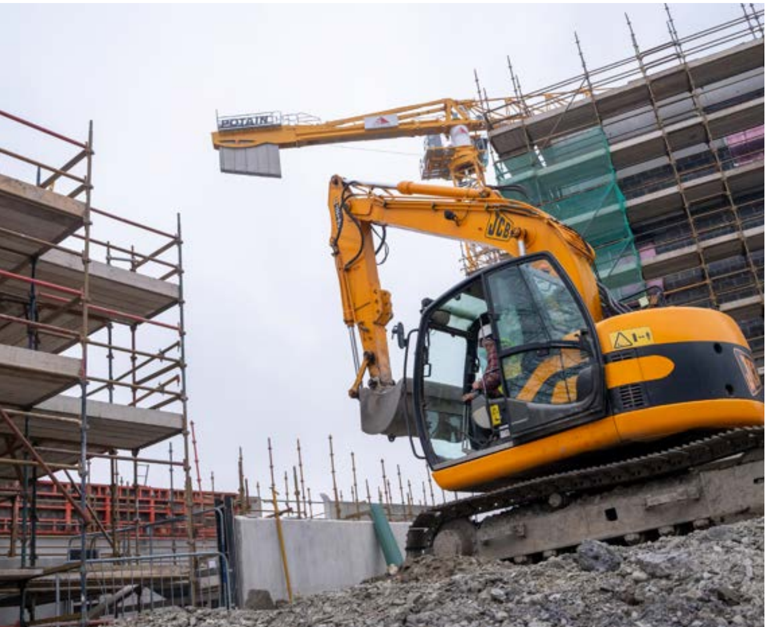
The school construction included 12% local employment over 2022. Image: Conor Mulhern
