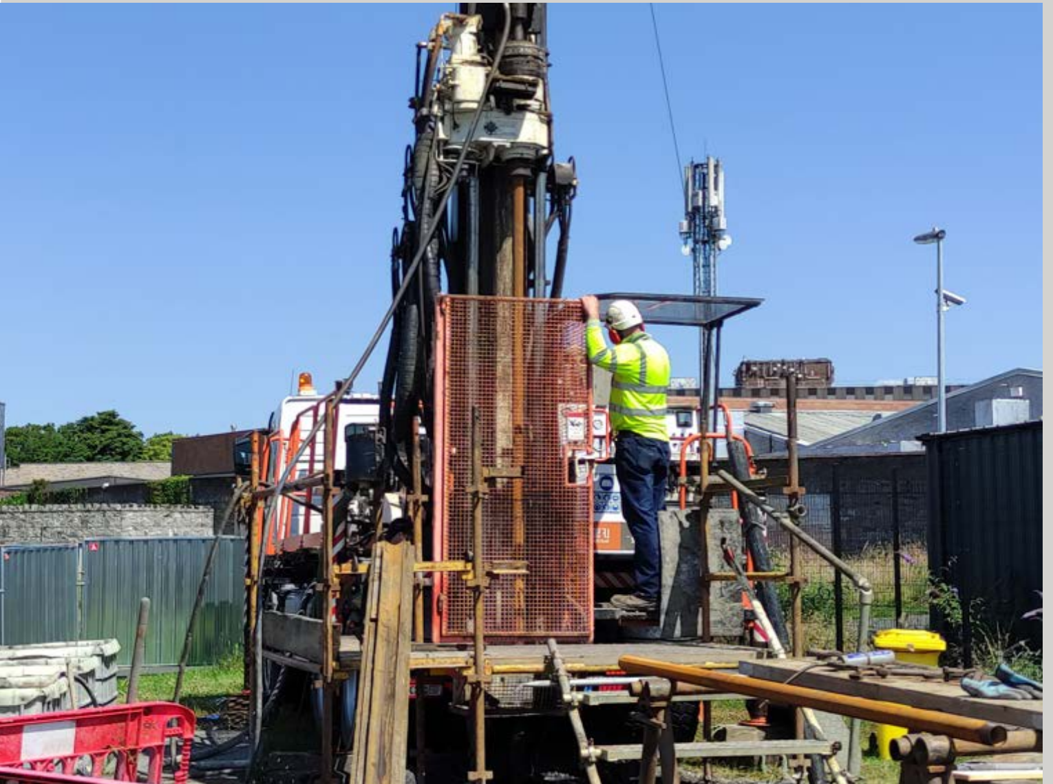
Initial exploratory borehole for geothermal on site, 2021. Image: Agency
