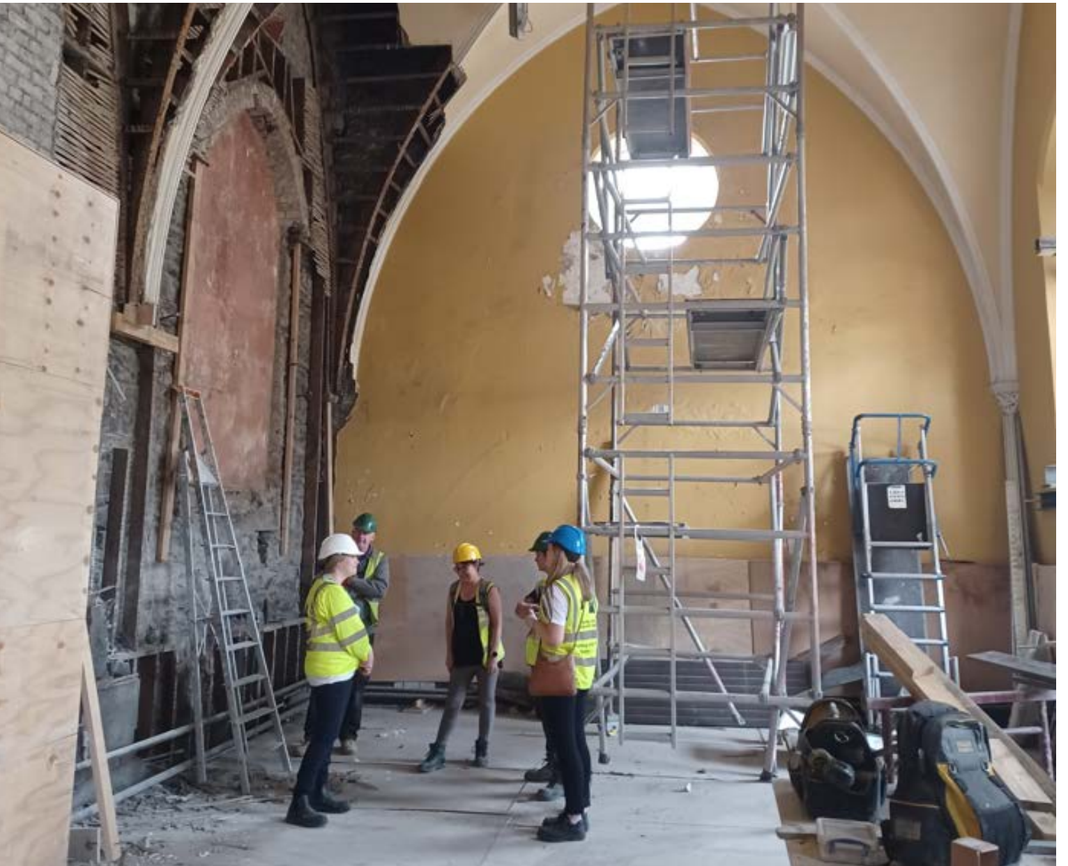
Clock Tower Stabilisation Works, DCC Visit. Image: Agency
