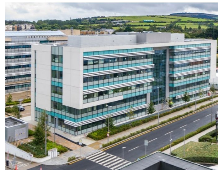
Vhi 360 Health Centre, Carrickmines
