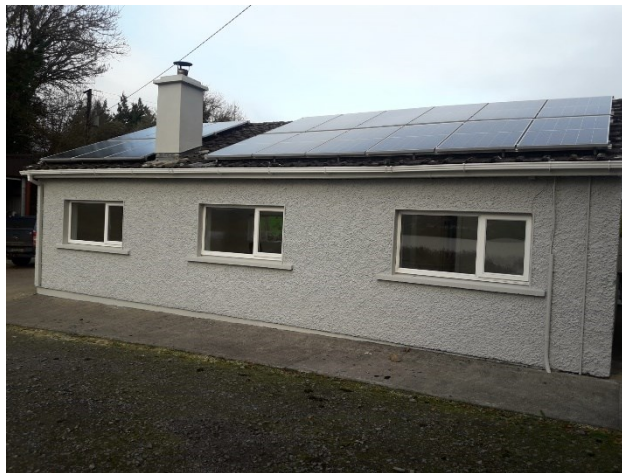
Image: Loch Arrow Base made energy efficient with solar panel roofing
