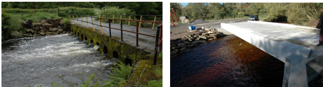
Images: Brook Lodge Bridge pre-works (left) and bridge under construction (right)
