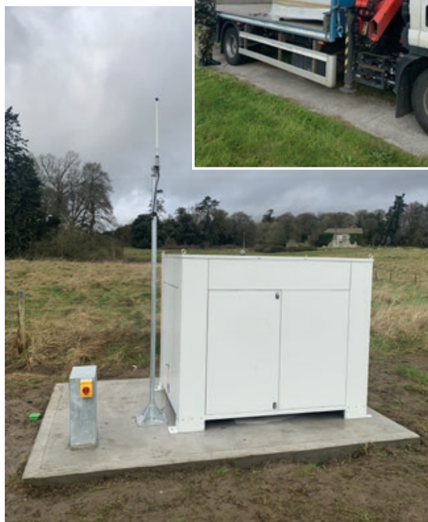
NRMN site at Athlone Barracks showing progression of work
