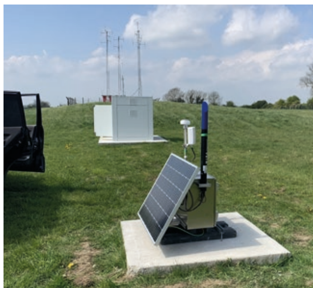
Onsite deployment of gamma dose rate monitor
