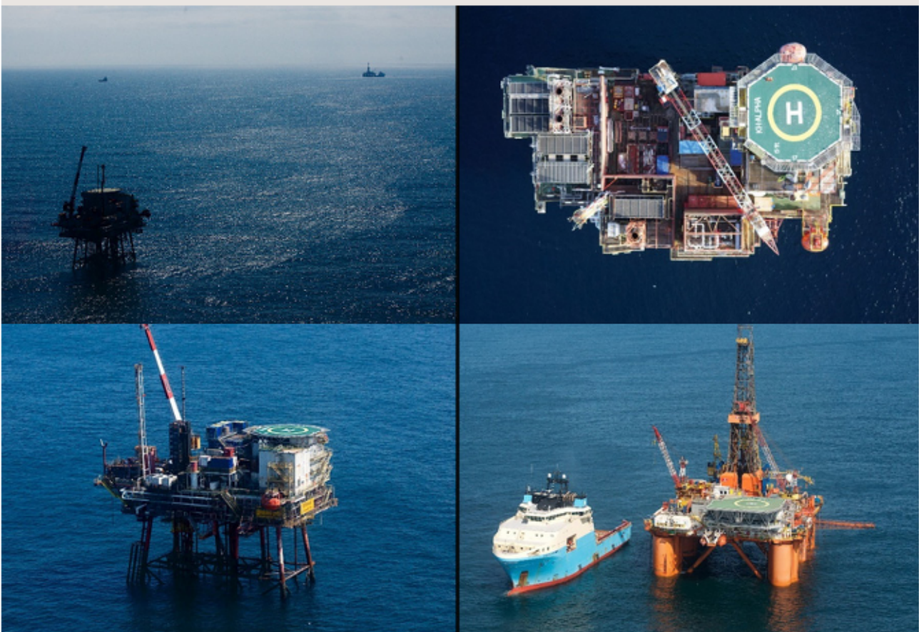
Figure: Alpha Platform & Bravo Platform (courtesy of KEL)
