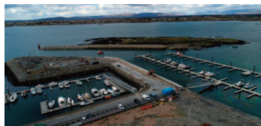
Breakwater Extension, Ros An Mhíl FHC Construction Contract Works completed in 2019
