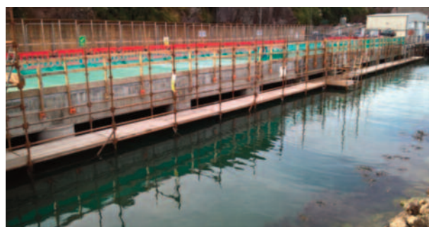
West Wharf Remedial Works Phase 4, Dunmore East FHC Construction Contract Works in progress 2019
