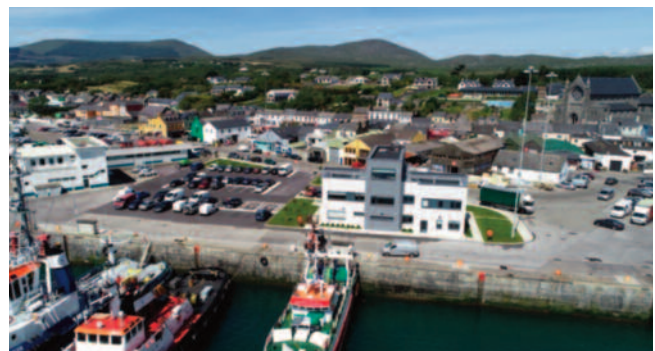
New Harbour Administration Building, Castletownbere FHC Construction Contract Works completed in 2019
