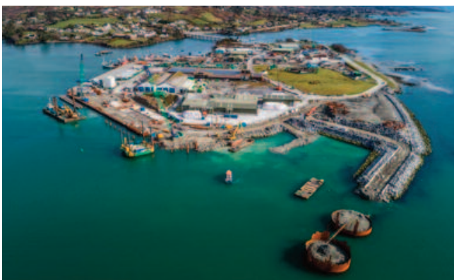
Dinish Wharf Expansion, Castletownbere FHC Construction Contract Works in progress 2019
