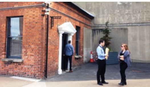
Pictured here is the refurbished Gatelodge building, opened in January 2014 to create additional space for The Digital Hub.
